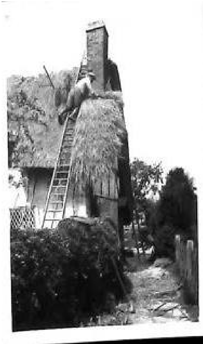
Re-thatching a cottage, about 1930. From a Walter Scott view pack. Thatchers worked on ricks as well as roofs: in 1851 two are counted among Welford's farm workers. 16/25
